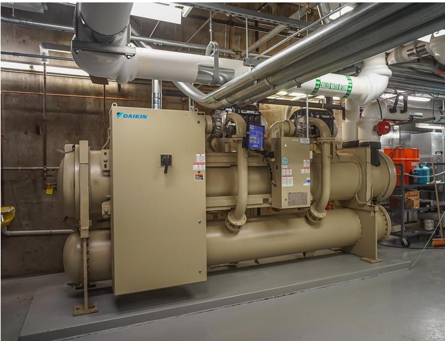
*Magnitude is up to 40% more efficient than standard centrifugal chillers and can save up to \$4 million over the life of the chiller. Facility managers can count on their chillers running at peak efficiency year after year with a design that wipes out the risk of contamination from efficiency-robbing oil buildup on to heat-transfer surfaces.*
