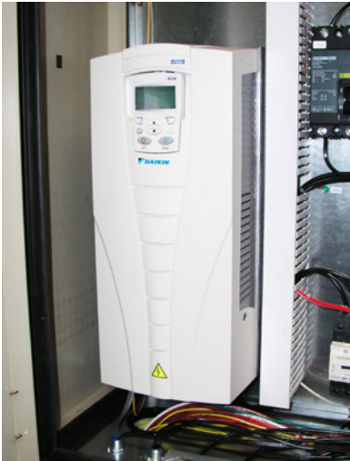
Figure 12: Variable Frequency Drive Controller
