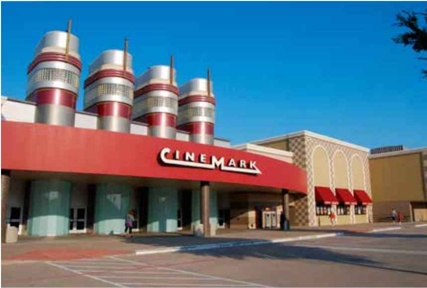
The Cinemark 16-theater cinema in Allen, Texas (near Cinemark headquarters in Plano) was used to test HVAC technologies.
