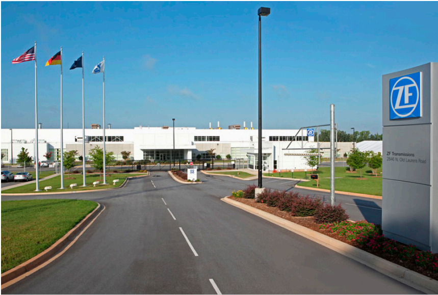
The ZF Transmissions facility opened in July 2013 and the new expansion is expected to be complete by 2016
