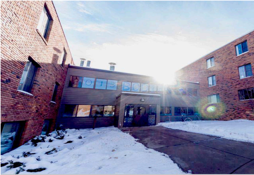
Two Bethel University residence halls faced dehumidification challenges due to showers, open doors, and a variable Minnesota climate.
