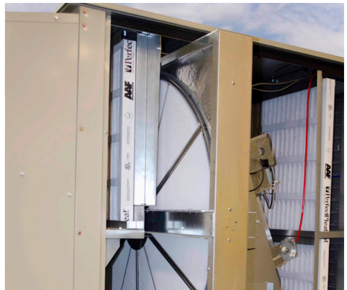
Rebel's energy recovery wheel draws 60% more humidity from the air stream for substantial energy savings and improved student comfort.
