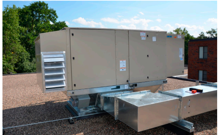
The 7-ton Rebel units deliver 20.6 IEER and use direct expansion and ERW technologies to maintain humidity comfort levels below 55%.
