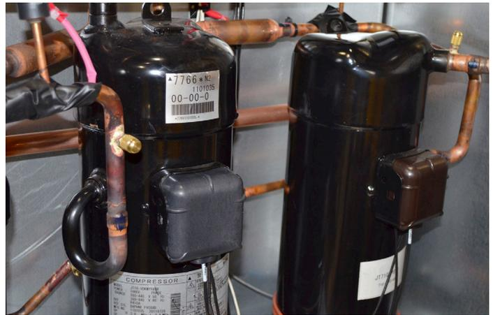
*Rebel’s modulating inverter scroll compressor allows for superior comfort control, energy efficiency, and cost savings than typical compressors.*
