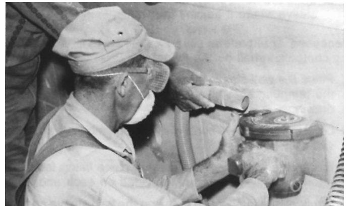
Figure 13: The interior wall opening is cut
