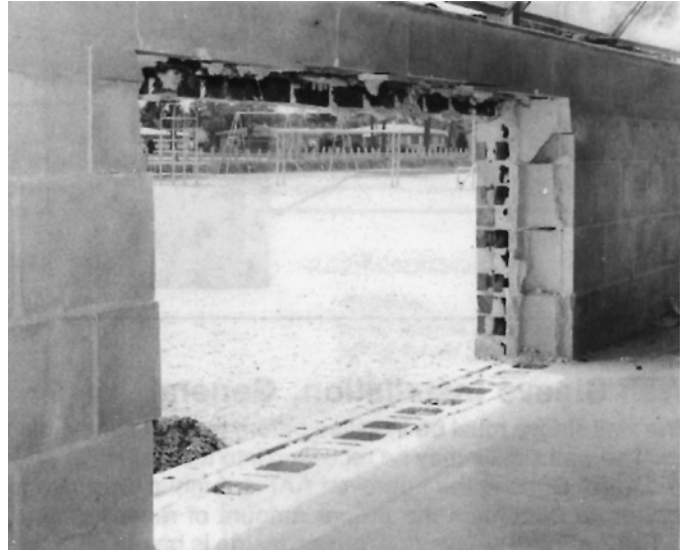
Figure 16: Lintels installed
