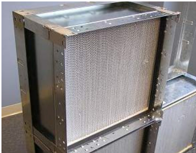
Figure 46: Properly Installed HEPA Filter
