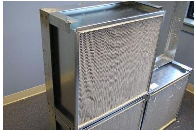
Figure 37: Filter Placed Inside of Frame
