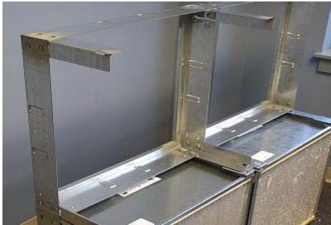
Figure 35: Frame with Leg Extensions Installed
