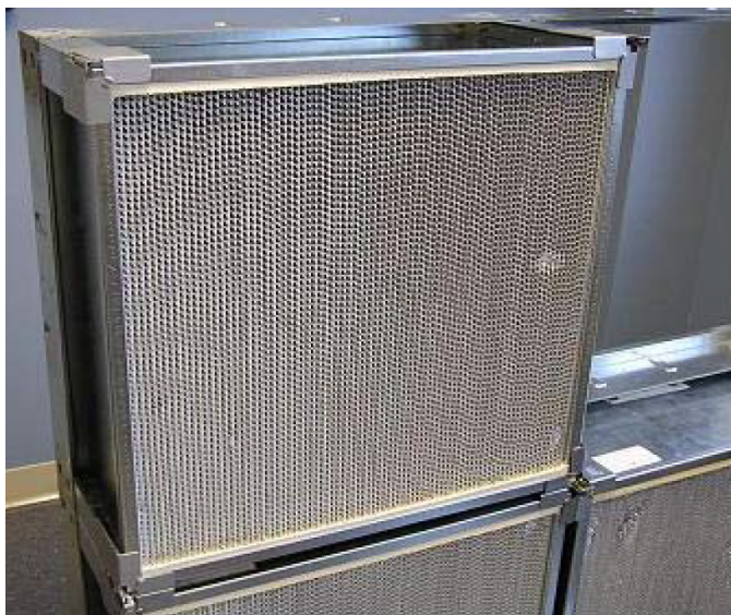
Figure 41: Properly Installed Filter Inside of the Frame
