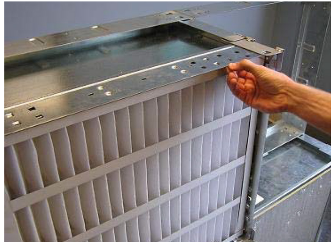
Figure 47: Installation of Prefilter into Frame
