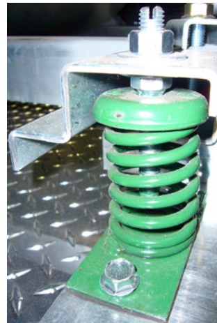
Figure 9: Spring Isolation
