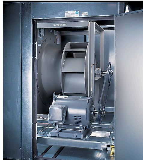
Figure 7: Plenum Fan
