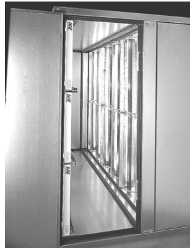
Figure 16: Attenuator Section
