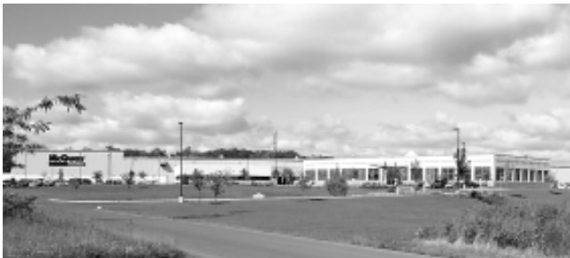
McQuay Air Conditioning plant with over 450,000 square feet of manufacturing space - located in Auburn, New York
